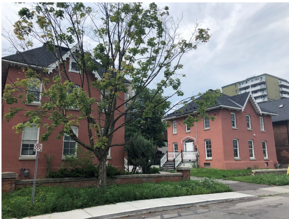
Photo 2: View of 283 and 285 McLeod Street, looking north.
