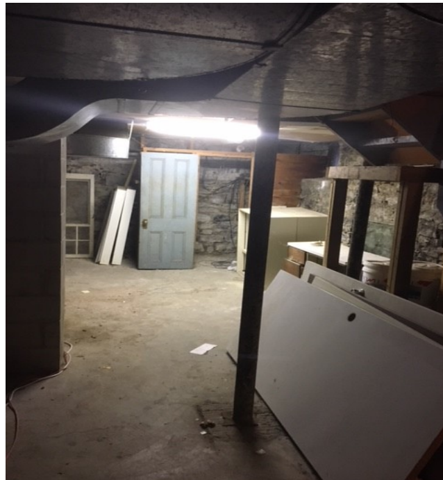
Photo 6: Typical Photo of unfinished stone foundation basement.
