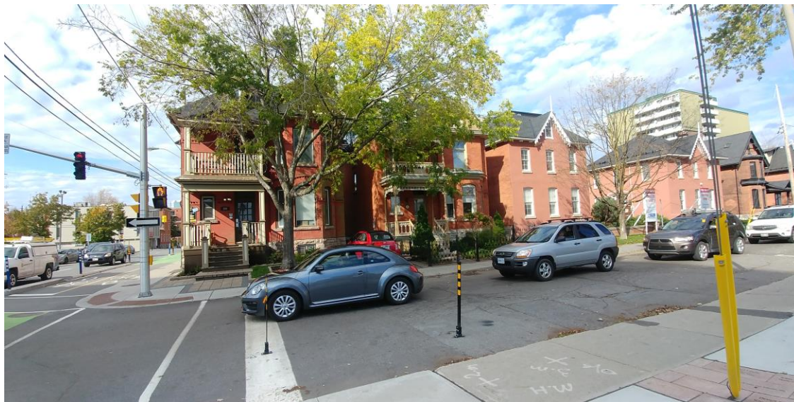
Figure 3: Context view looking northwest at the intersection of Metcalfe. The 12-storey high-rise framing the block at O'Connor and Gladstone is very visible. The 8-storey unit directly behind the subject property is not intrusive from this view. Source: Google Maps
