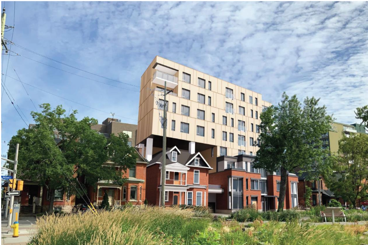
Figure 20: A view looking north-east with the proposed mid-rise set behind the two units on the street. Source: grc Architects 2021
