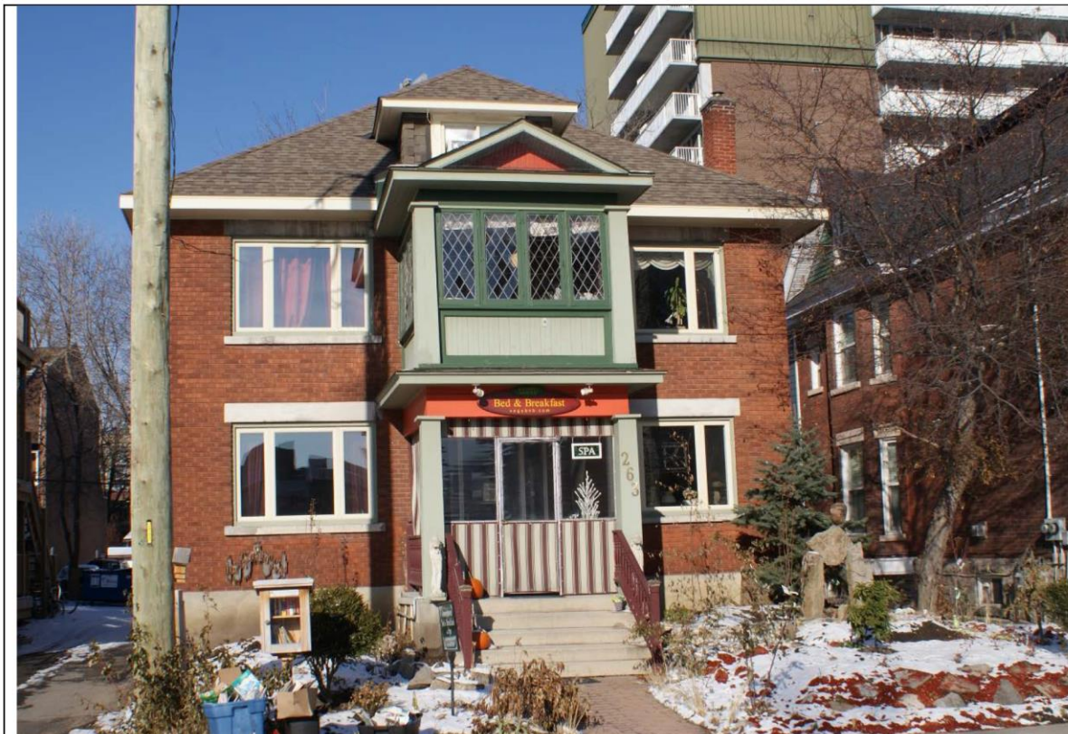
View of 263 McLeod Street which was constructed during the same time period 1925-46 as the building at 283 McLeod.
