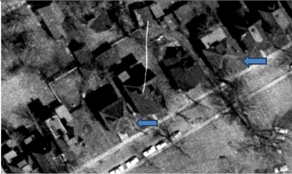
1965 Aerial view of McLeod with 283 McLeod (left) and 263 McLeod (right) both arrowed. Note the four-square plans with similar hip roofs and entrances fronting onto the street with porches.
