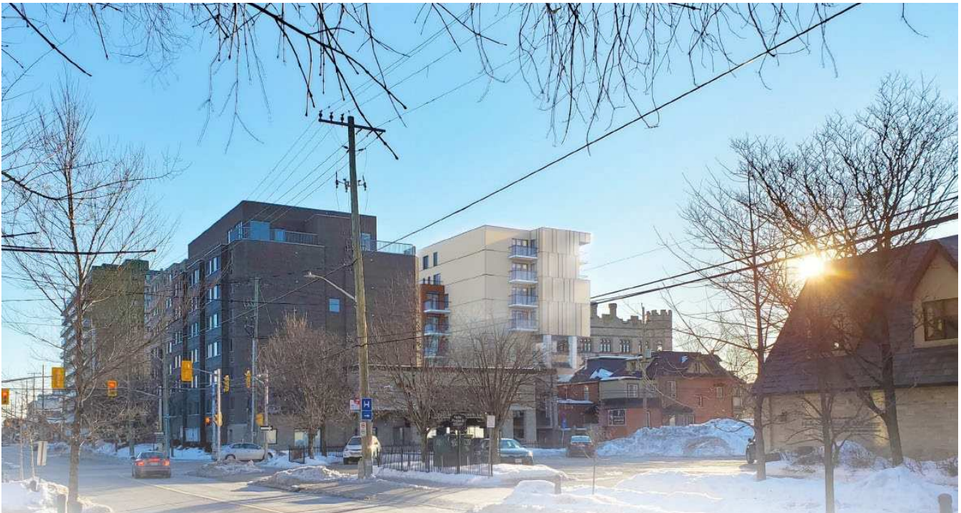
Figure 22: Looking southeast towards the proposed development from Gladstone Avenue
