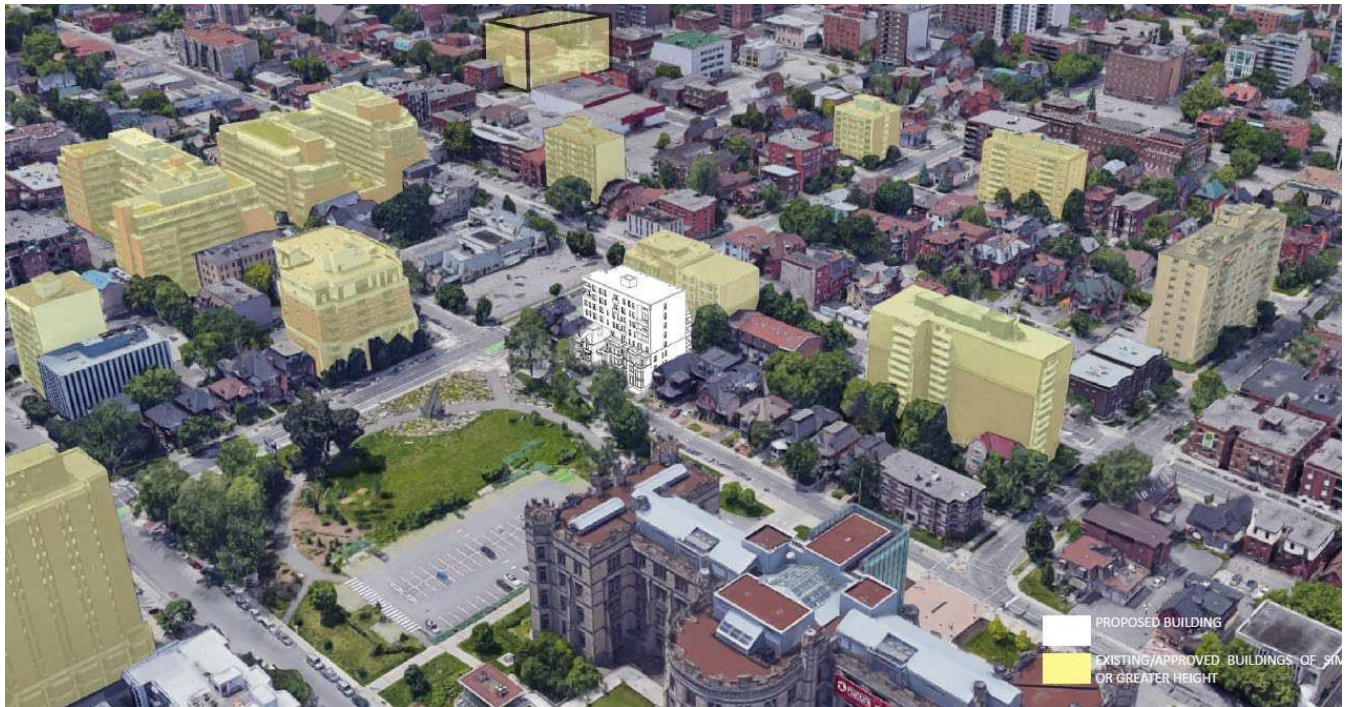
Figure 12: Looking northwest to the proposed development within its context, subject site in white, mid-rise buildings indicated in yellow
