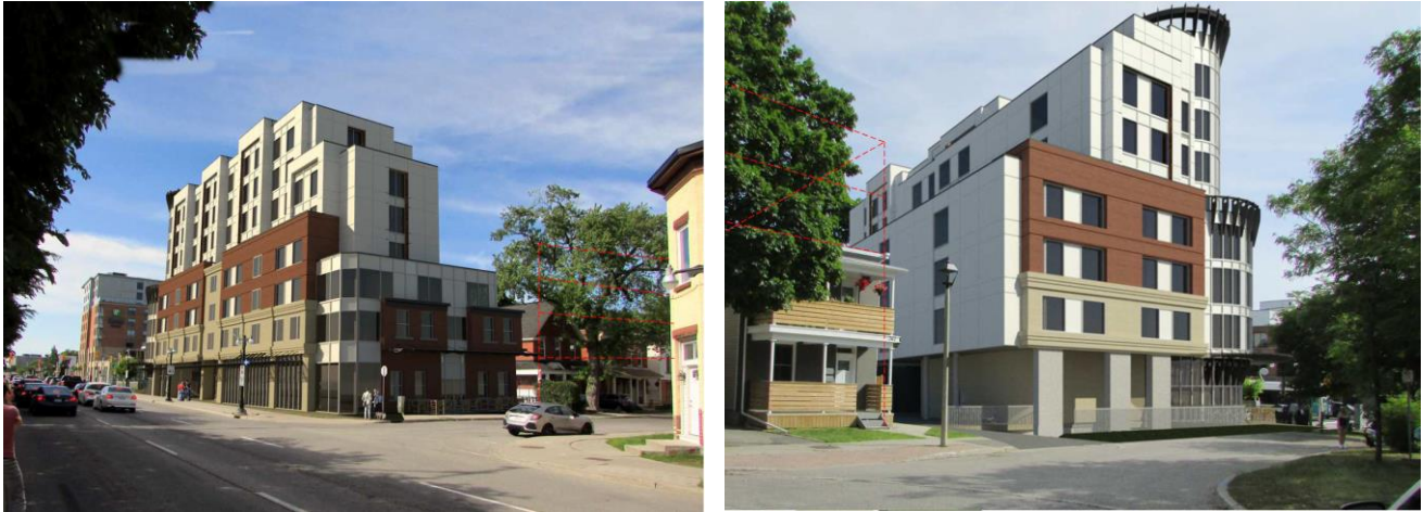
Figure 14: Two views highlighting the revised plans with the additional corner property. Source: Woodman Architect & Associates 2021.
