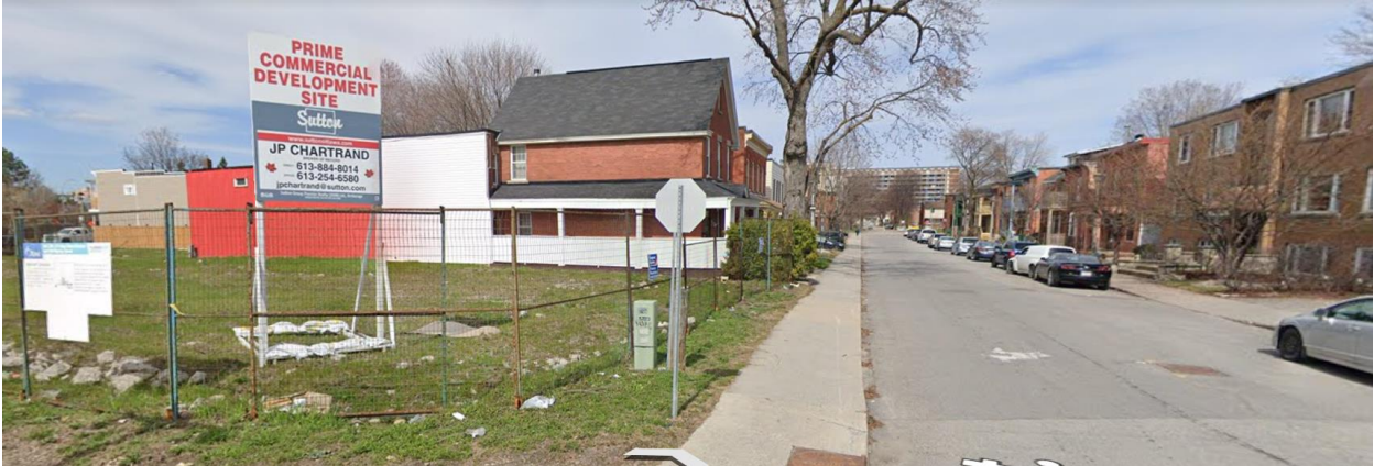
View of the Property looking east along Clarence Street.
