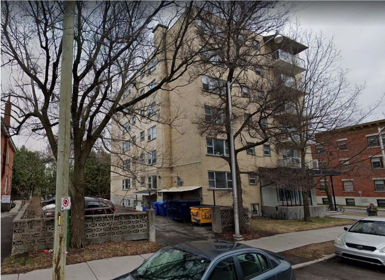
Figure 2: Existing building located on the subject property
