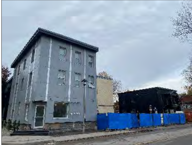
Photo 3 – Site Building (east elevation).
