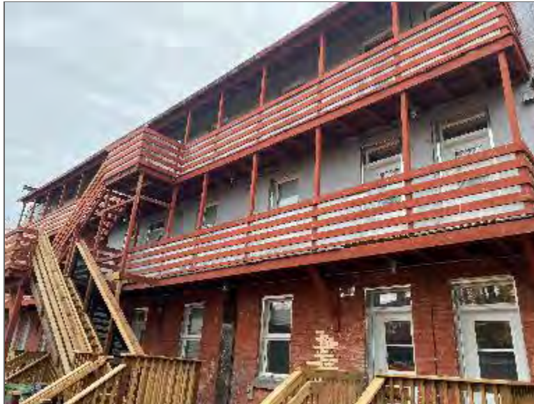
Photo 1 – Site Building (partial north elevation).
