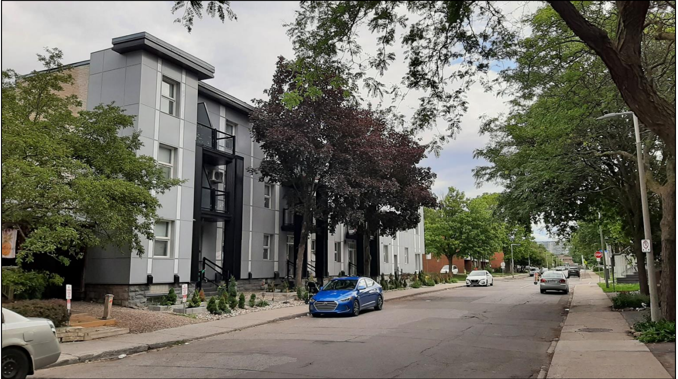
Figure 5: Subject site shown with two mature trees in the front boulevard
