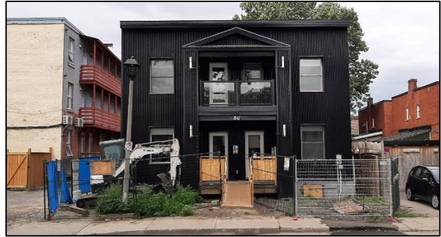
Figure 20: Looking west toward the existing Nelson Street building
