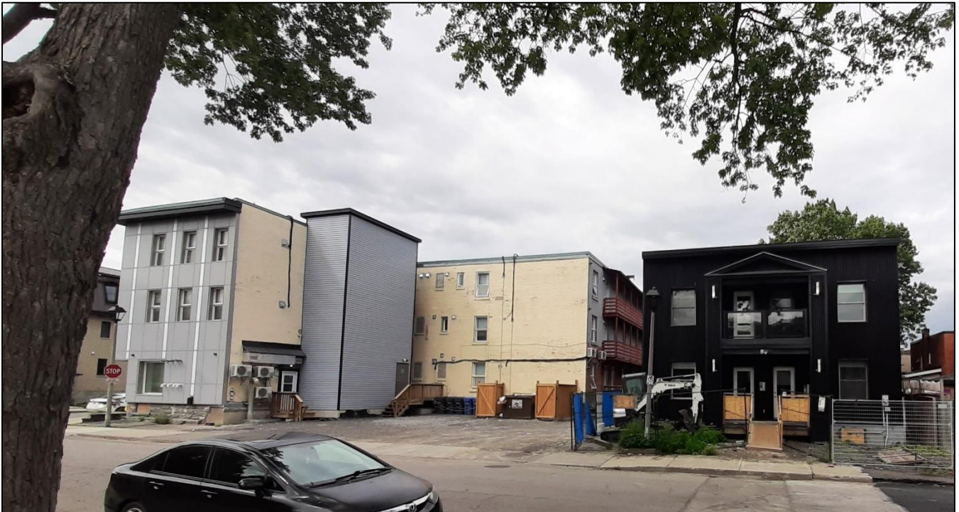
Figure 23: Existing east frontage of the subject site
