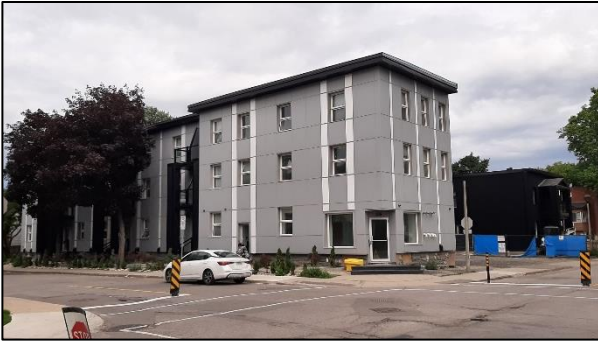
Figure 19: Looking northwest toward the subject site with the York Street building prominent in the foreground and the Nelson Street building visible in the background
