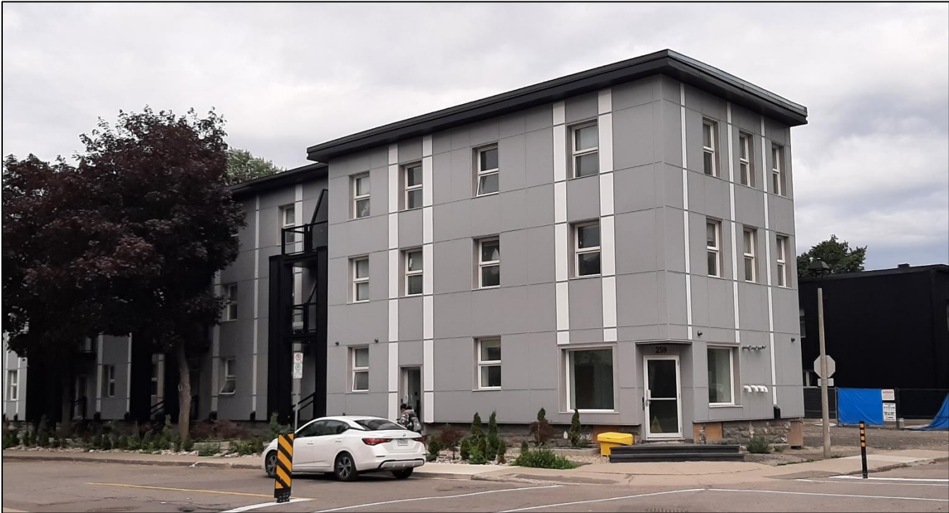
Figure 2: Subject site with 253 York Street shown in the foreground
