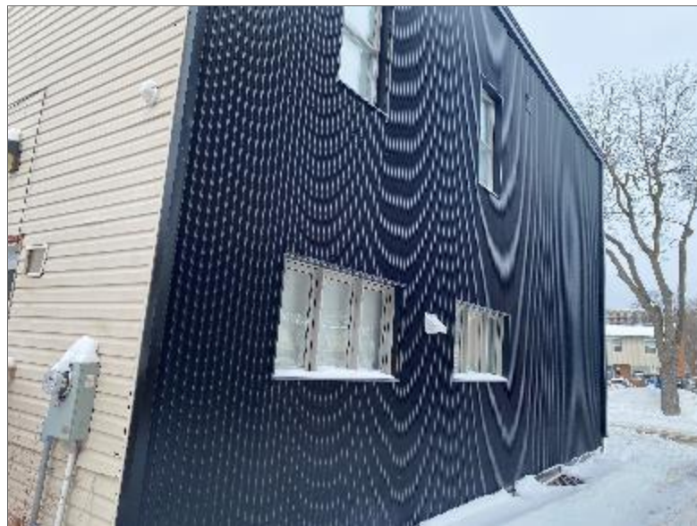
Photo 4 – Site Building B (south elevation).
