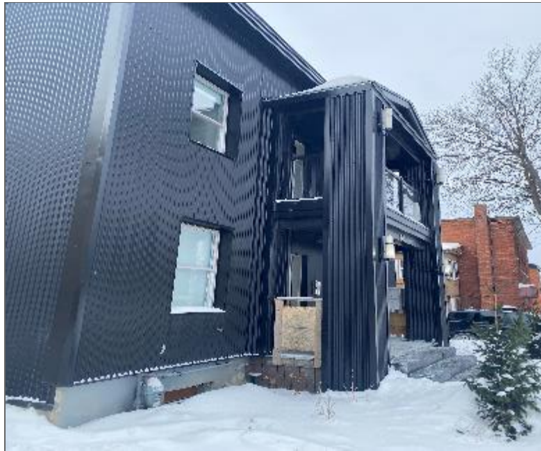
Photo 3 – Site Building B (east elevation).
