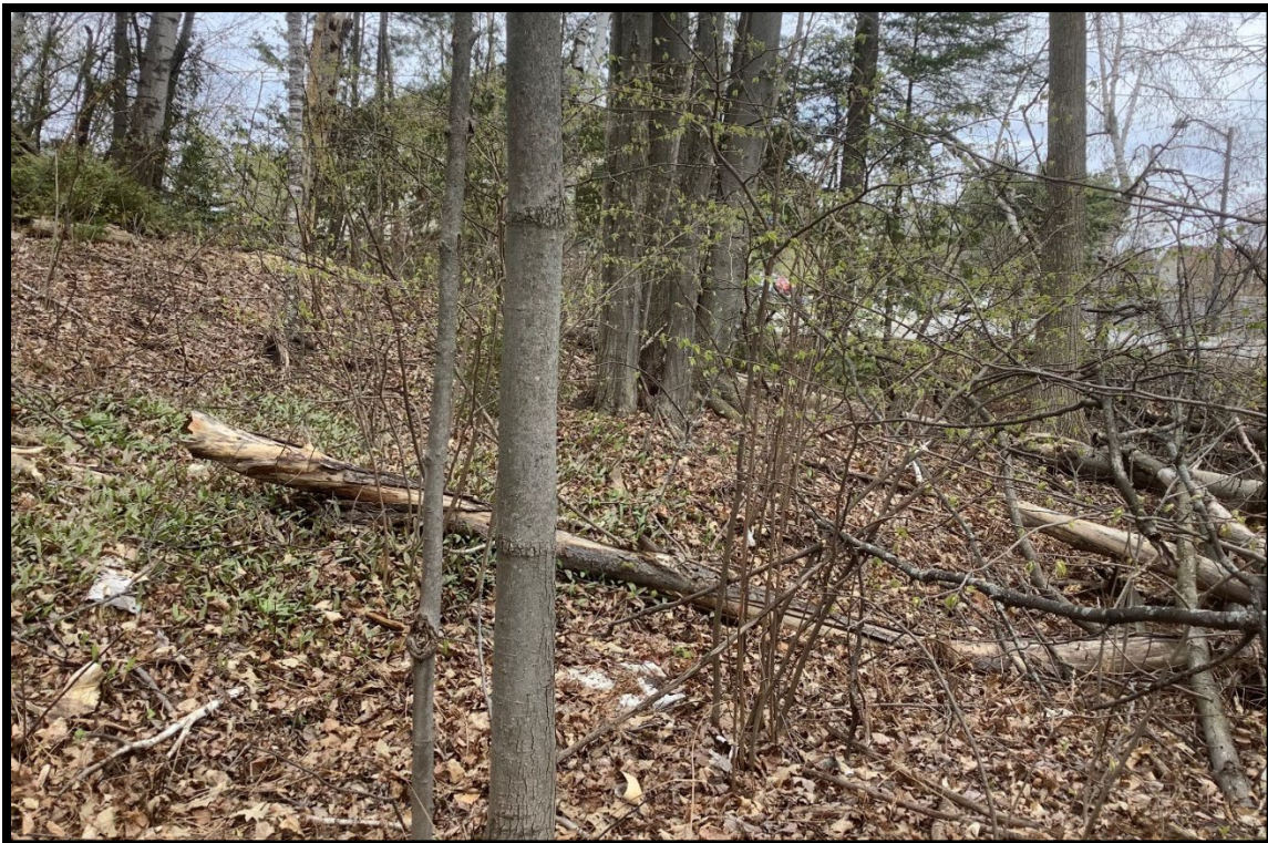
Figure 2: Rise from fill along eastern edge of forested part of study area (D56).
