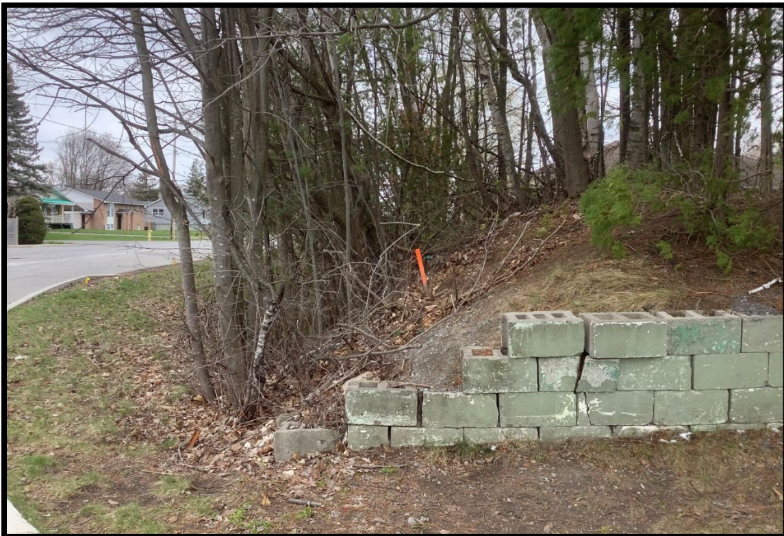
Figure 12: Concrete block retaining wall holding up fill along Pagé Road (D50).
