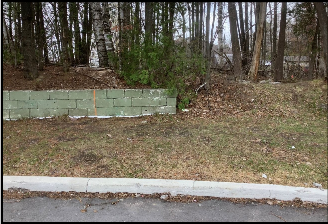
Figure 13: Concrete block retaining wall holding up fill along Pagé Road (D48).
