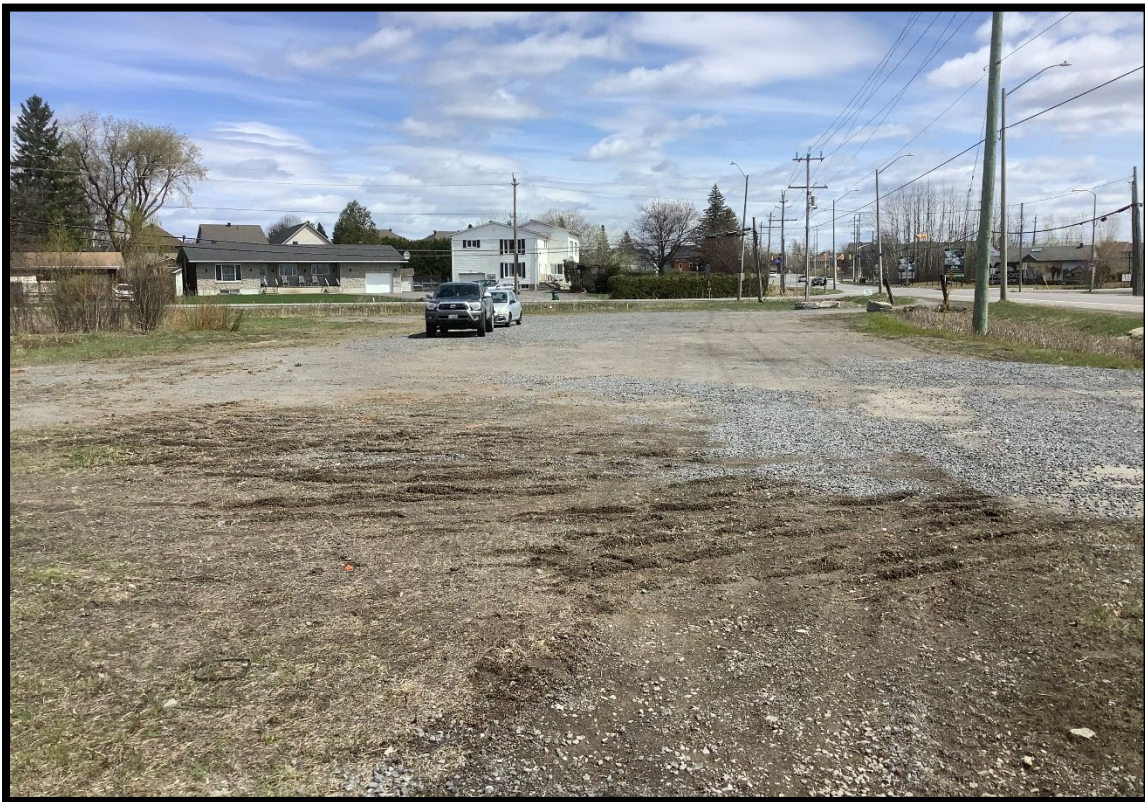
Figure 4: Gravel driveway and parking lot, looking towards intersection Navan and Pagé Roads (D05).
