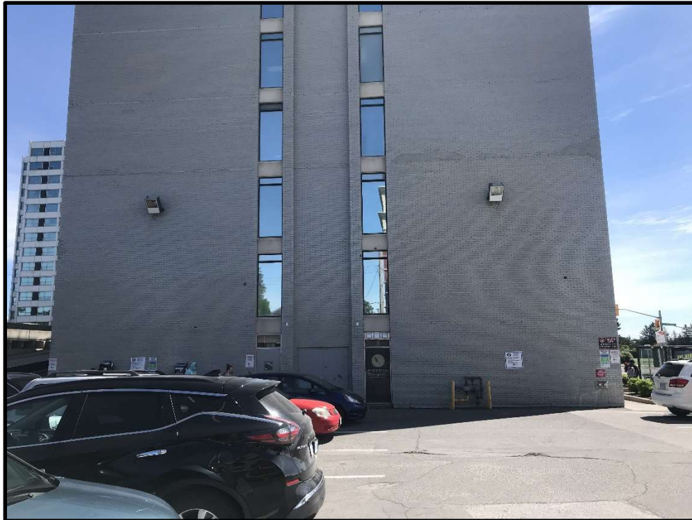
Photograph 2: West view of subject building, looking east.
