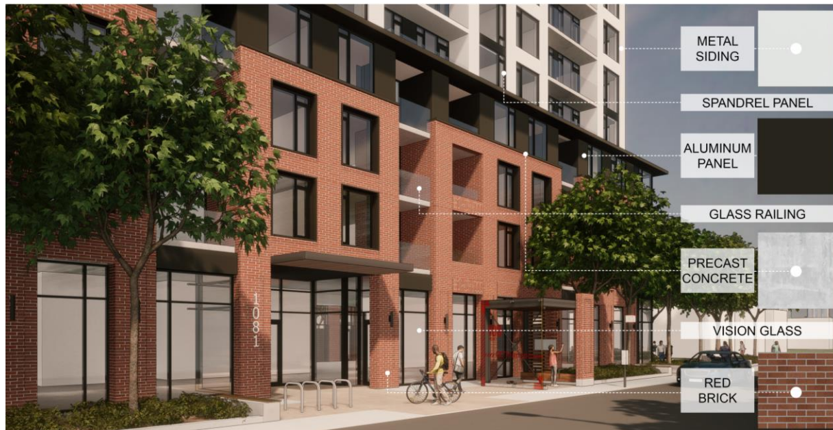
Figure 26: The developments material palette features a red brick podium with established datum lines that reference nearby buildings. Source: Hobin Architecture 2022.
