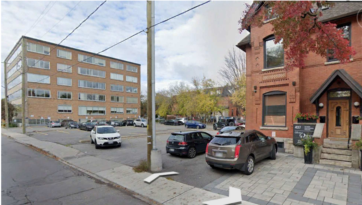
Figure 3: Street view looking north-west across the parking lot at 359 Kent. The heritage property at 437 Gilmour forms the eastern edge of the proposed development (left). Source Google Earth
