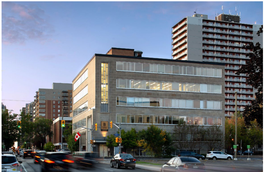
Figure 2.0 – Existing Legion Building at 359 Kent Street.
