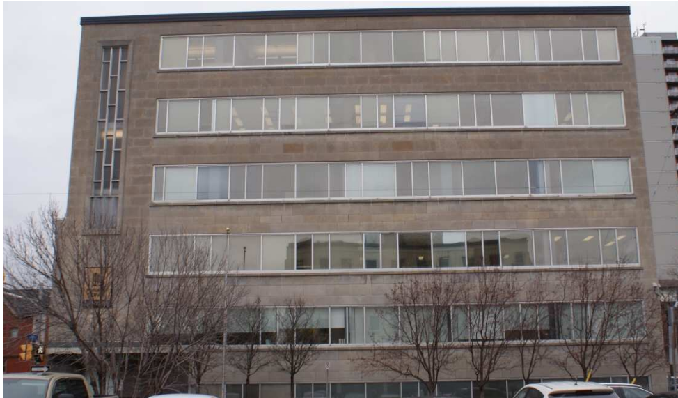
Figure 30: View of the windows on the Gilmour Street façade. All of the original windows have been replaced with the exception of the three-storey window above the Gilmour Street entrance. Source: Commonwealth 2022.
