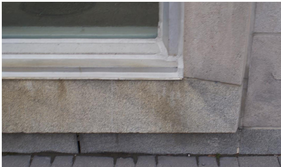
Figure 18: Detail of the granite plinth course and granite windowsill surround at the base of the three-storey Kent Street window. The colour of the granite sill is very close to the limestone cladding and window surrounds. Source: Commonwealth 2022.
