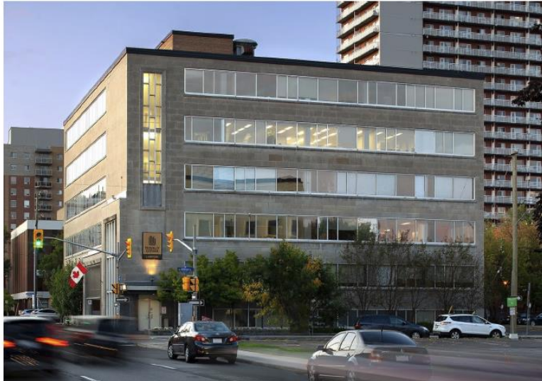
Figure 2 - Current condition, 2022, of Legion House
