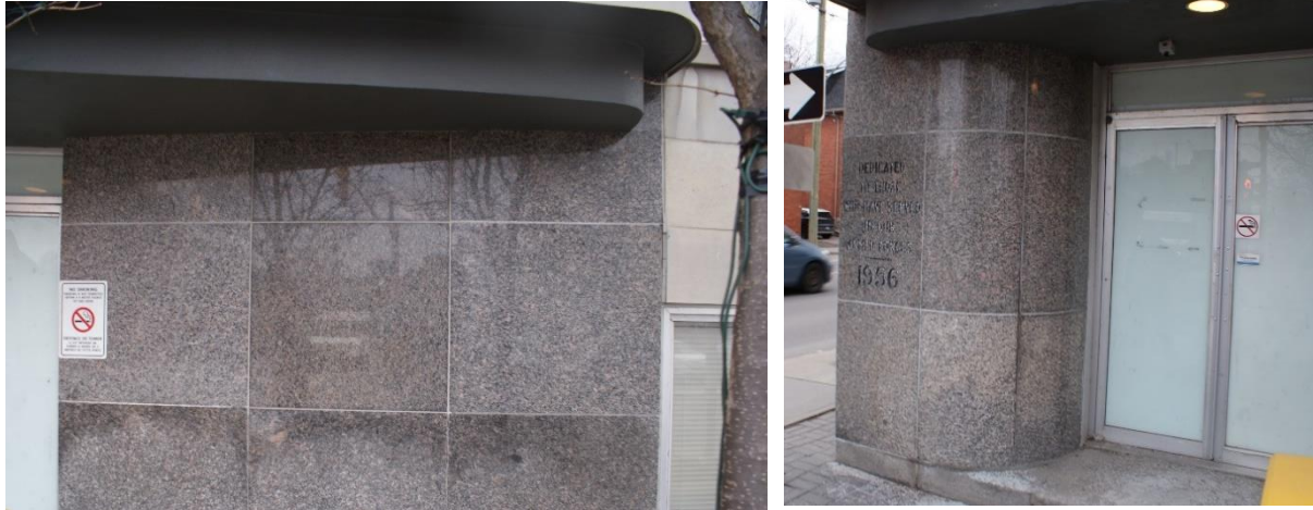
Figures 10 & 11: (6 -left) View of the introduced polished granite panels to the right of the Gilmour Street entrance. (7-right) View of the original polished granite panels. Source: Commonwealth 2023
