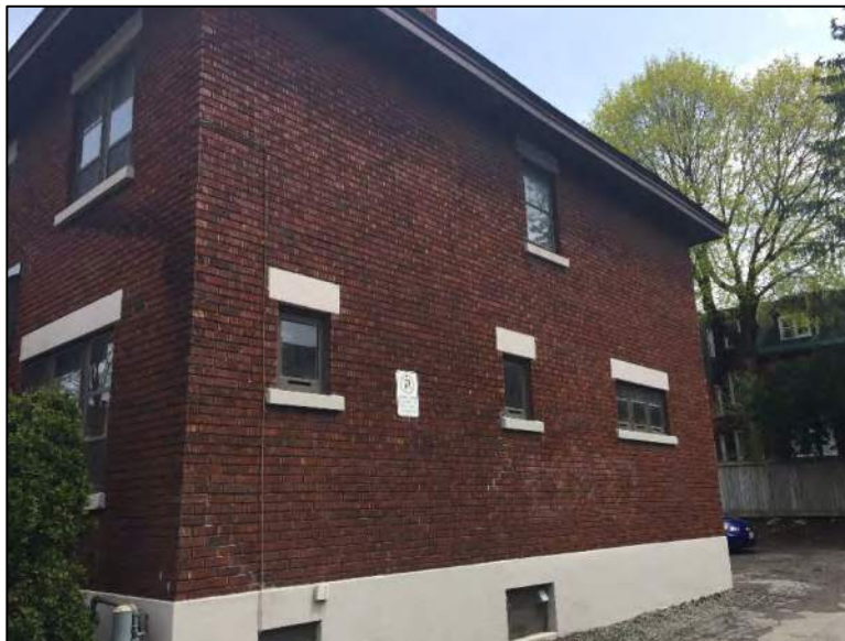
Photo 4 – Site Building (west elevation).
