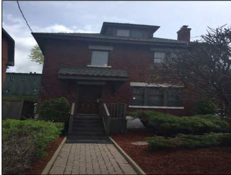
Photo 1 – Site Building (north elevation).
