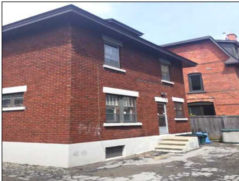
Photo 2 – Site Building (south elevation).
