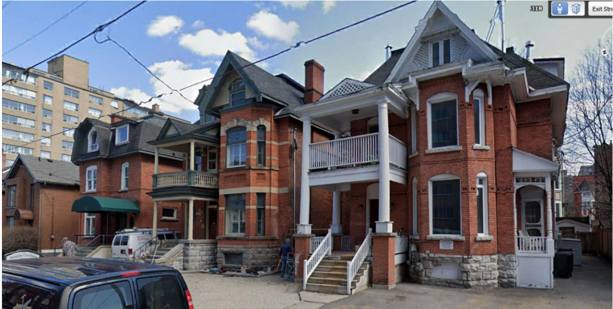
Figure 5: Contextual streetscape view of properties to the east of the development site that illustrate the built context on the south side of Waverley Street. Source: Google Earth
