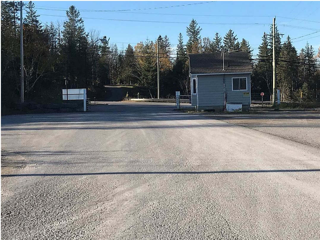
View of Existing Quarry Access to March Road
