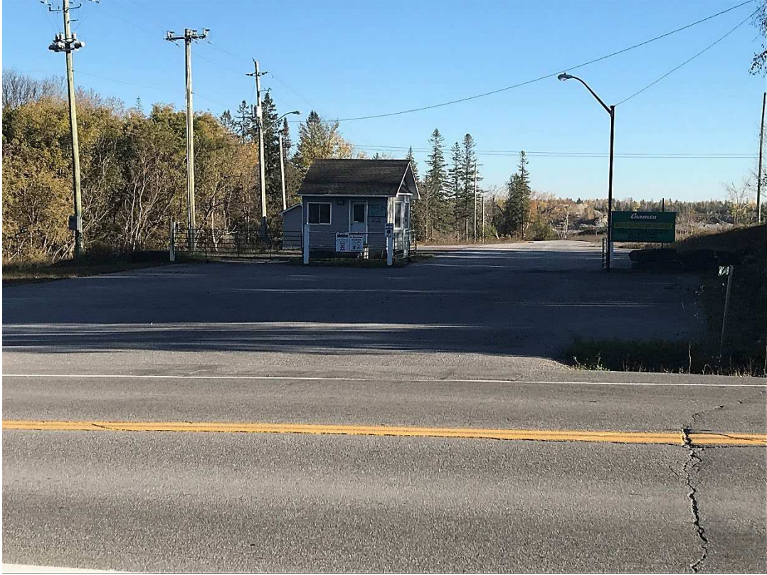
View of Existing Quarry Access from March Road
