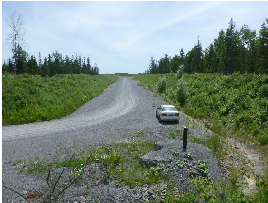
Image 5: Disturbed area showing gravel roadway and large berms facing southwest.
