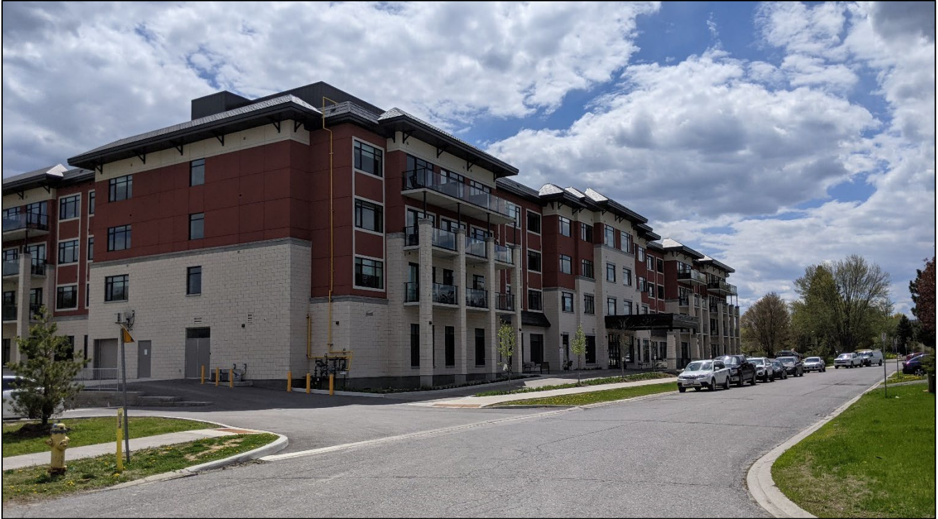
Figure 5. View looking southwest showing the Wildpine Retirement Living Centre.
