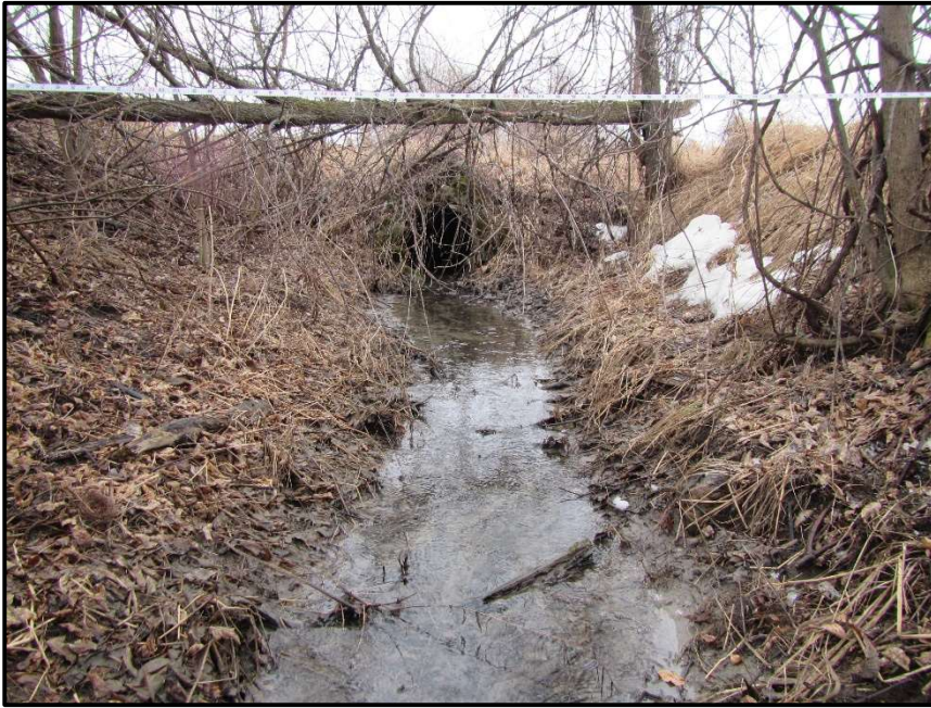
Photograph 5: Survey Site #3 downstream, facing upstream (March 24 th , 2021).
