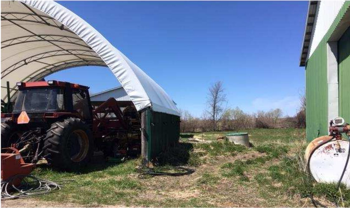
Photograph 2: View of the outbuildings (eastern and northern buildings), exterior diesel AST, domestic well and farm equipment, looking north.
