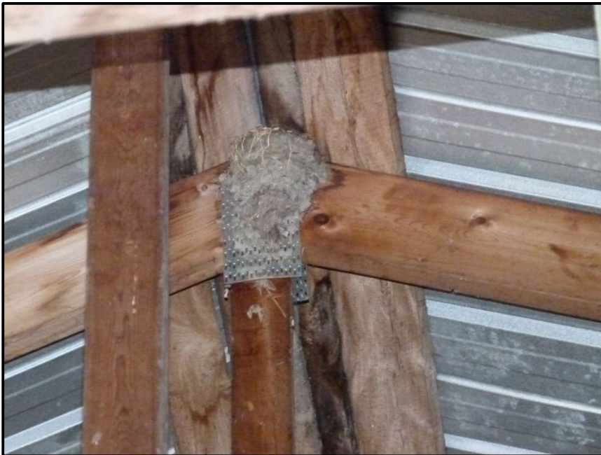
Photograph 20: Active Barn Swallow nest within Structure #2 (July 29 th , 2020).
