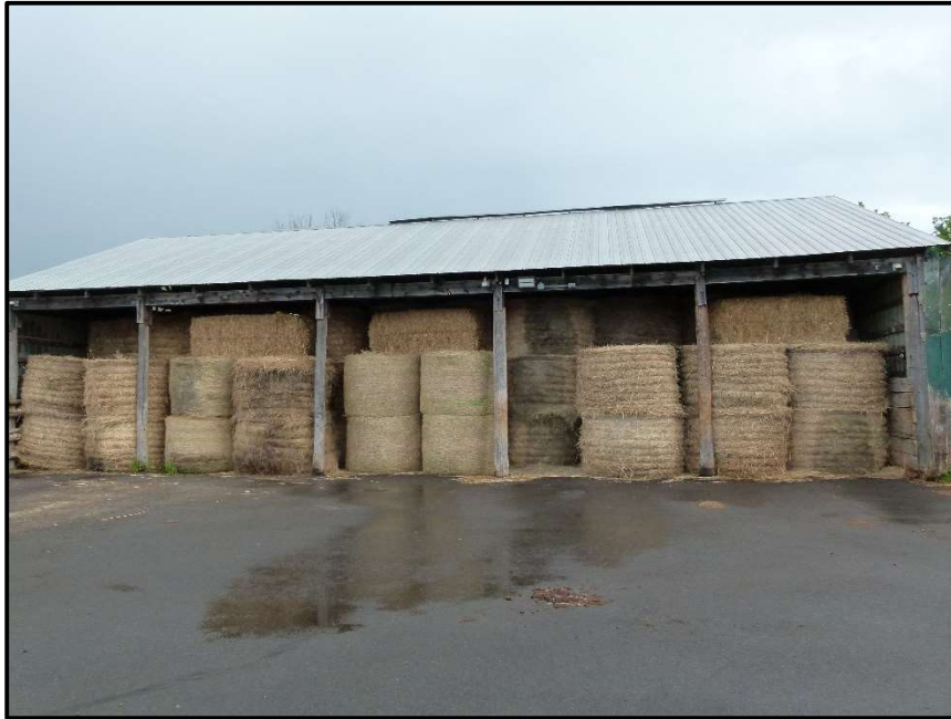
Photograph 23: Structure #5 (Hay Storage Area). One (1) Barn Swallow nest was observed within Structure #5 (July 29 th , 2020).
