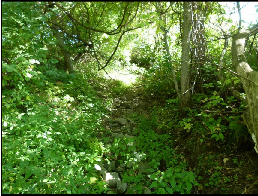
Photograph 14: Looking south at the northern end of the remnant portion of Drainage Feature C (September 17 th , 2020).
