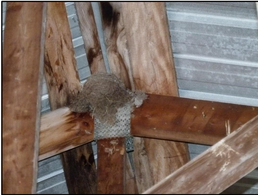
Photograph 19: Active Barn Swallow nest within Structure #2 (July 29 th , 2020).
