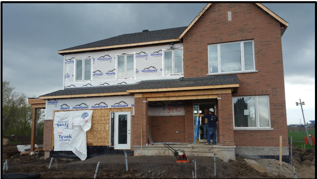
Photograph 4: View of the model home on the northern portion of the subject site, facing southeast.
