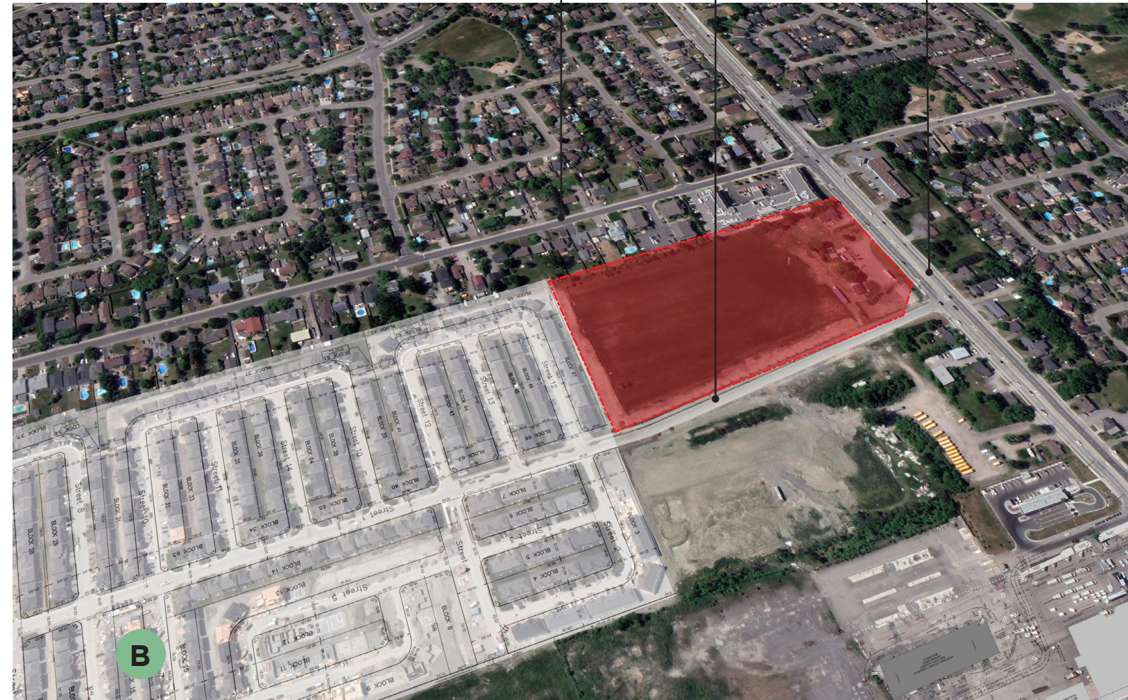
VIEW TOWARDS PAGÉ ROAD
