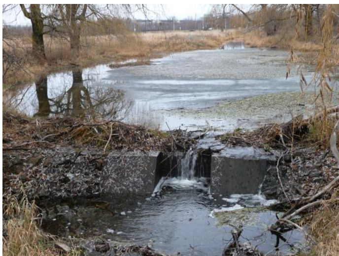
A weir constructed along Stillwater Creek downstream of Moodie Drive that was observed in 2009 and 2015
