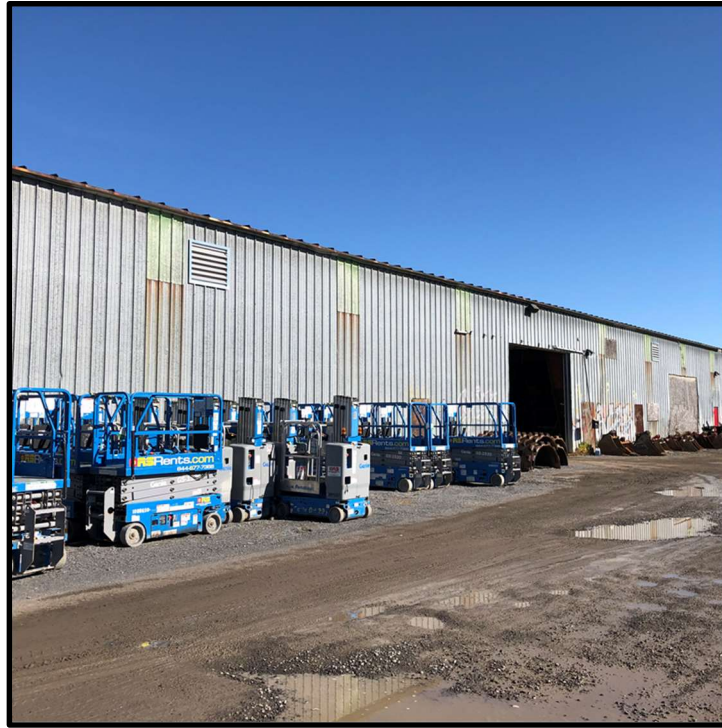
Photograph 1: View of subject building looking north.
