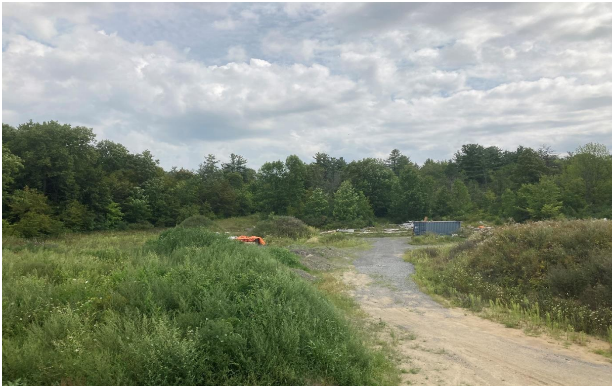
Photograph 4: North view of the subject site, showing a sea can and construction storage on site.
