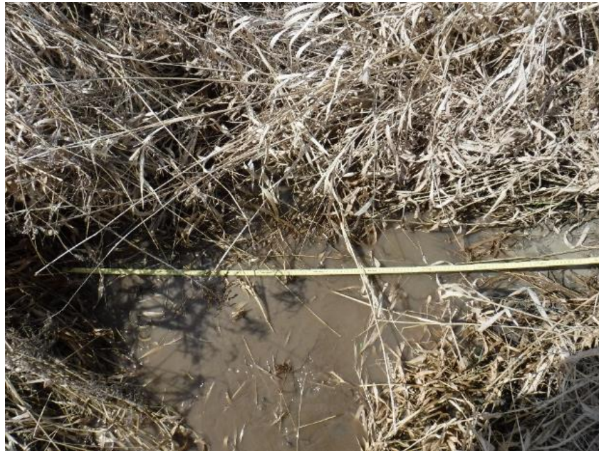
Photo A Downstream end of channel (vegetation was manually removed to allow for measurements) (March 30, 2021)
