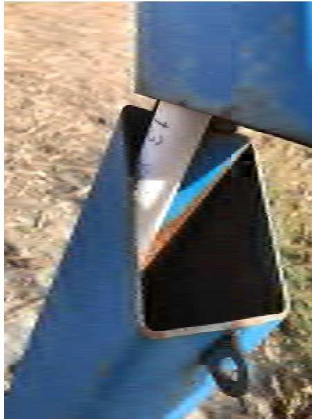
Photo 27 – Two of two existing, damaged wells at 4375 McKenna Casey Drive.
