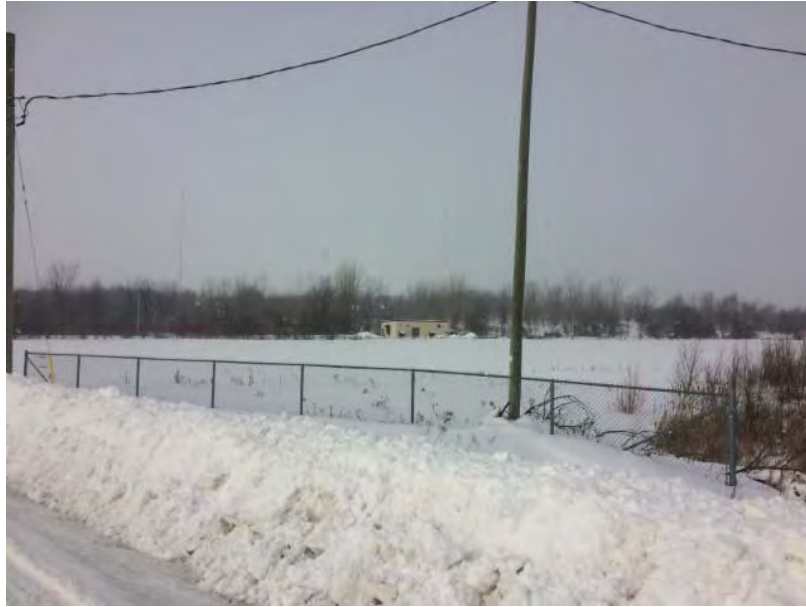
Photo 1 – Looking northwest at the cell towers and communications building located northwest of the Site
