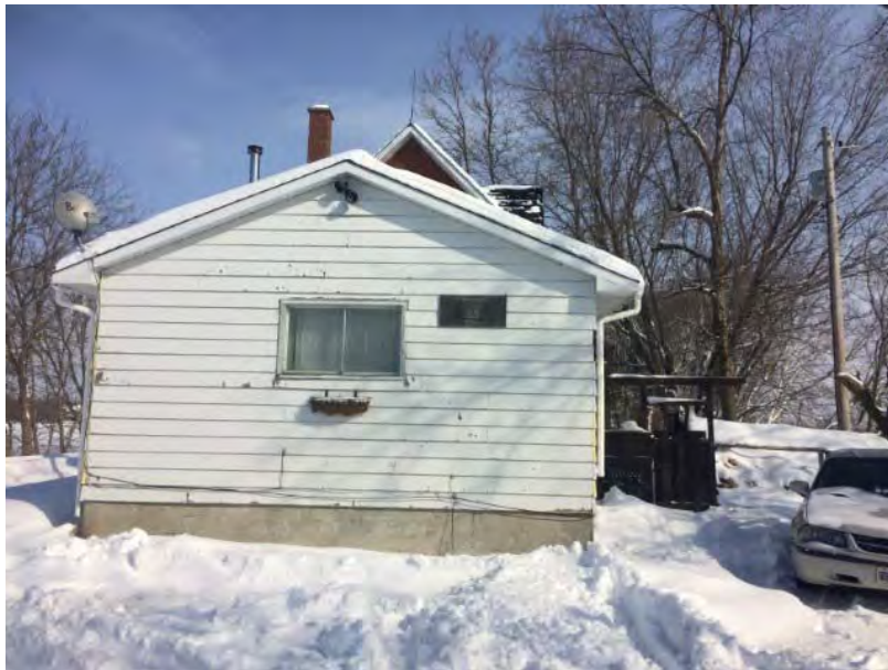
Photo 12 – Photo of the west side of the on-Site farm house
