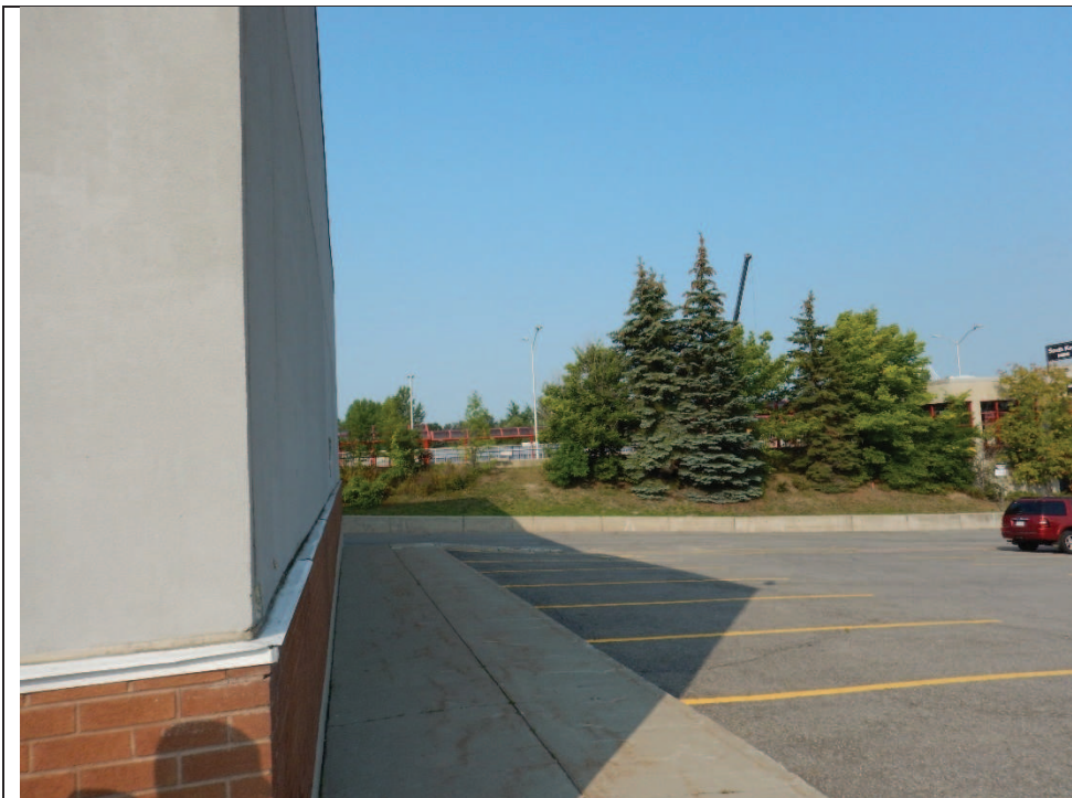
Photo 20: View of the west side to the Phase One Property including the OC Transpo Transitway (facing west) - 2021
