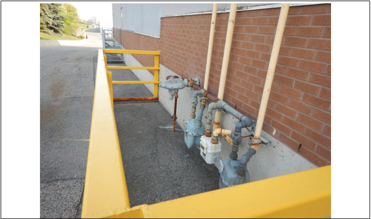
Photo 11: Natural Gas service for the vacant commercial retail space on the Phase One Property - 2021
