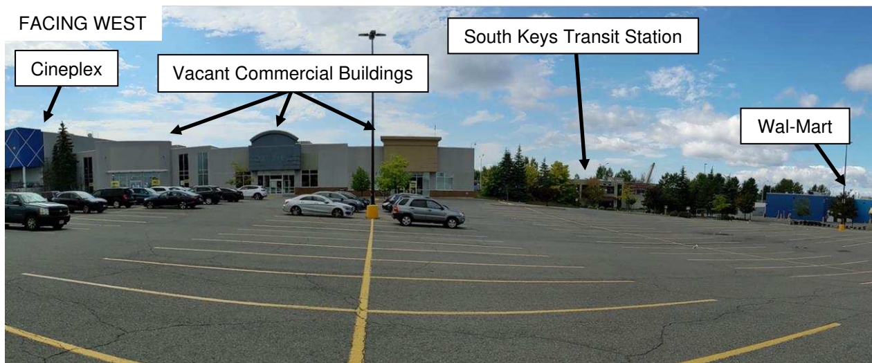
FIGURE 5. SITE CONTEXT PHOTOS (SEPTEMBER, 2021)
