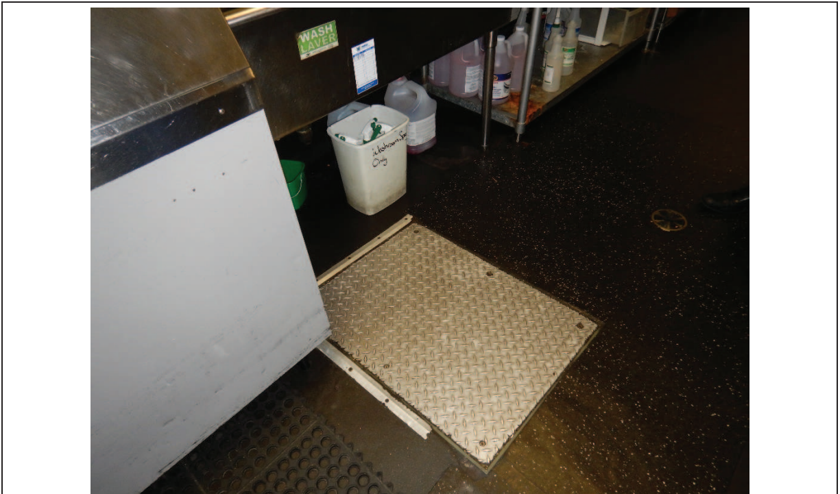
Photo 19: View of the grease trap in the Cineplex
