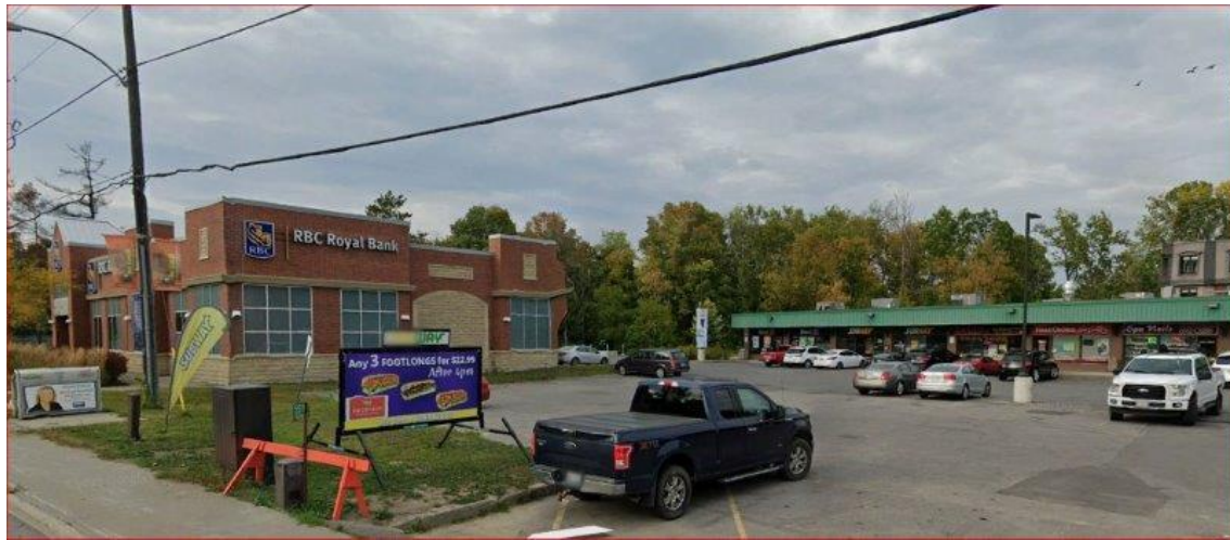
View of neighbouring mall South of the 5497 Main Street property
