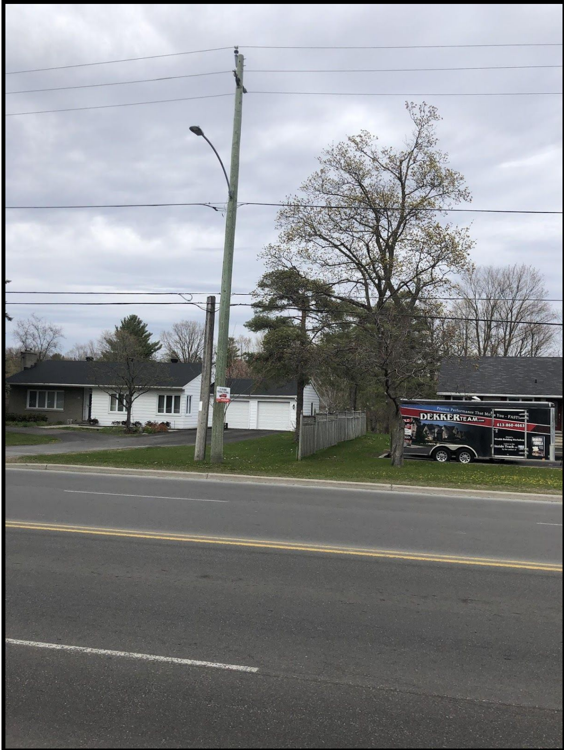
View of the front of the property (north half) taken from Manotick Main Street.
