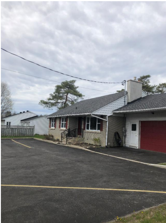
View of front of existing house
