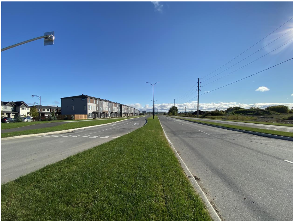
Figure 6: The existing road conditions and public realm of Campeau Drive.
