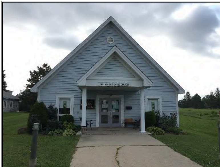
Photo 2 – Site Building A (west elevation).
