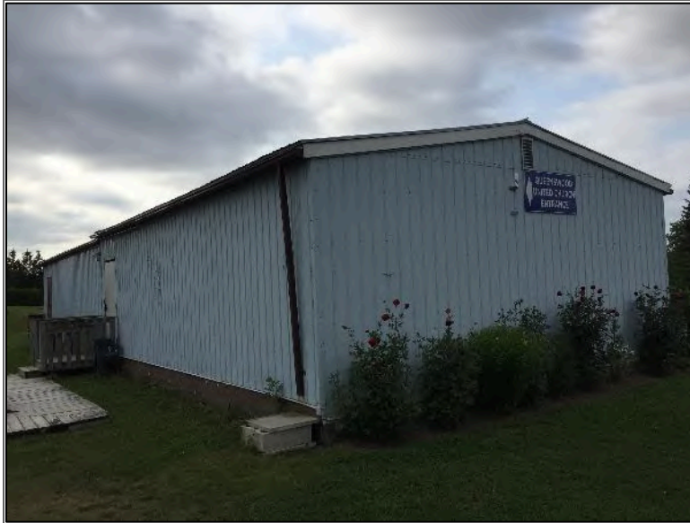
Photo 3 – Site Building B (north and west elevations).
