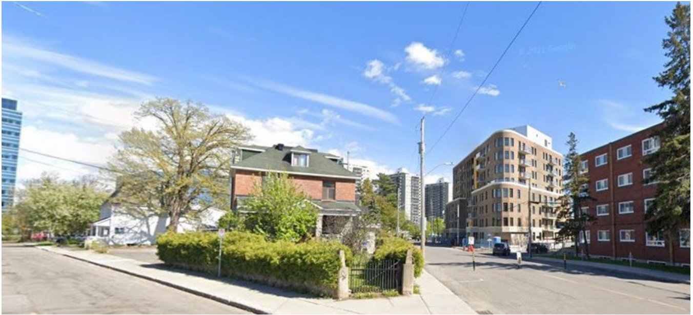
Figure 4: Subject Property looking east (existing buildings to be demolished).
