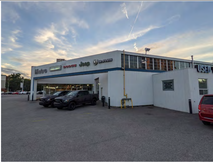
Photo 9 – Eastside of the building, facing southwest
