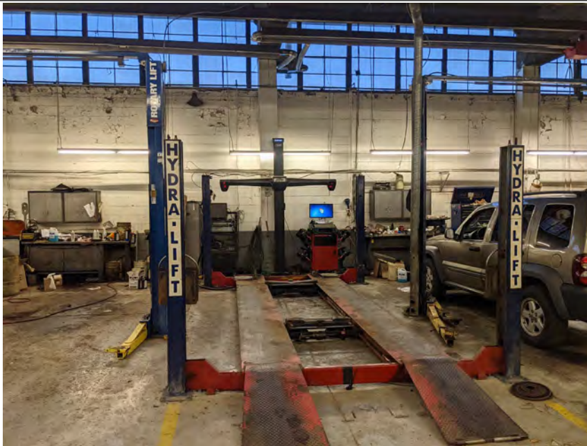
Photo 17 – Hydraulic hoist, located in the southeast side of the garage
