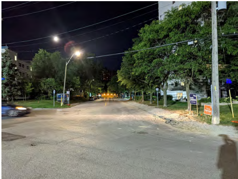
Photo 32 – Looking down Ambleside drive to the southwest
