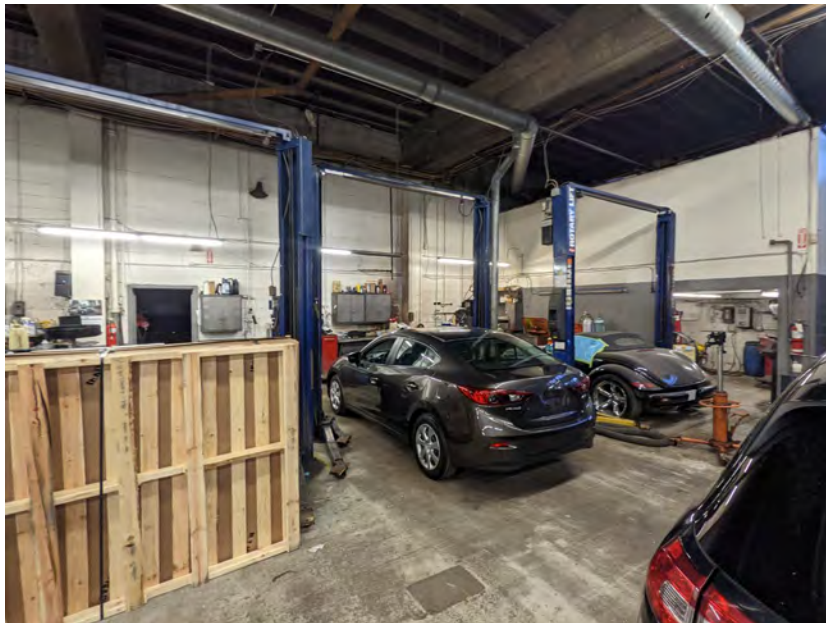
Photo 24 - Hoists in the garage, along the westside
