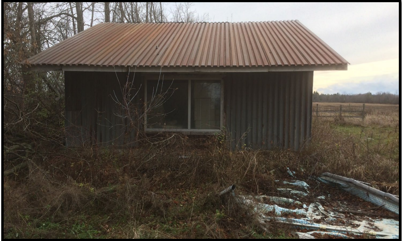
Figure 5: Shed behind residence at 1015 March Road. (PA1156-D34)
