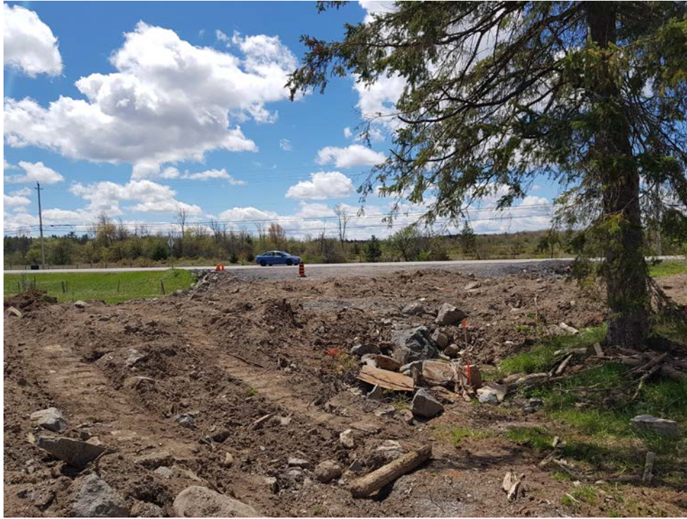
View of some fill materials used in roadway
