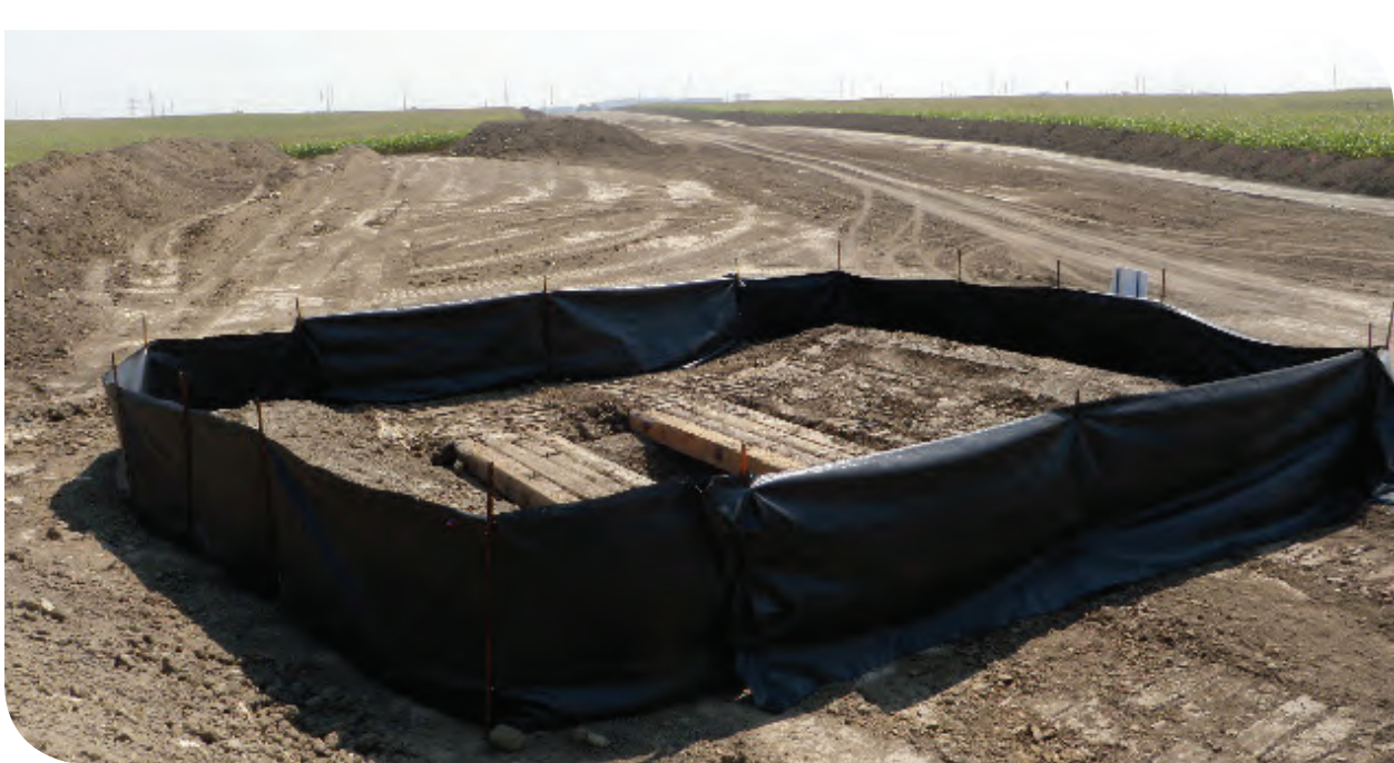
Cleaning station at construction site.
