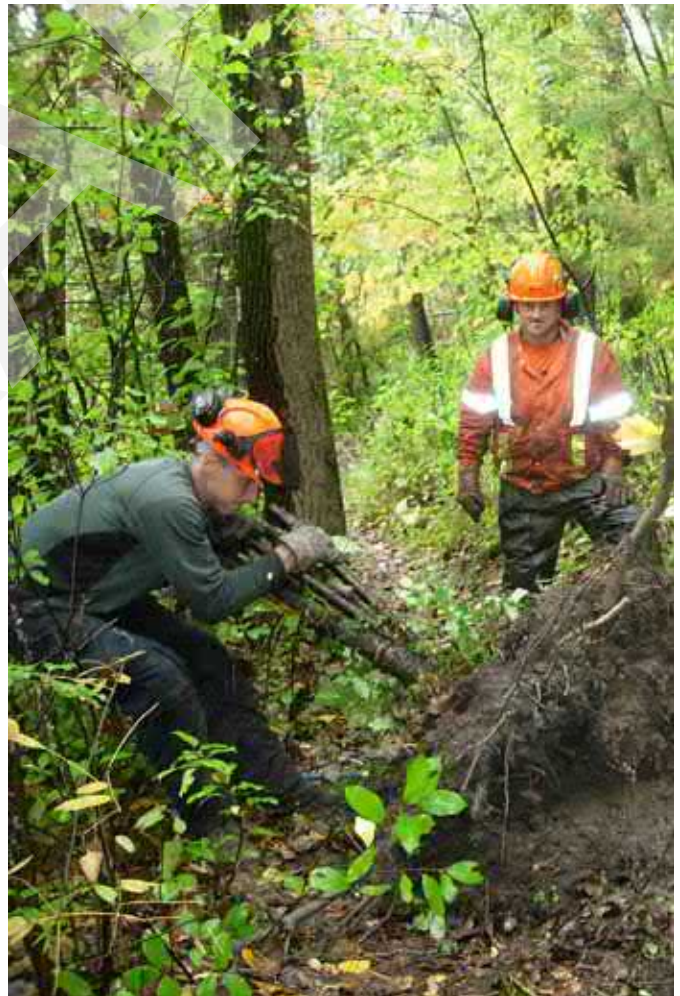
Removing a cut stump Photo courtesy of Iola Price.
