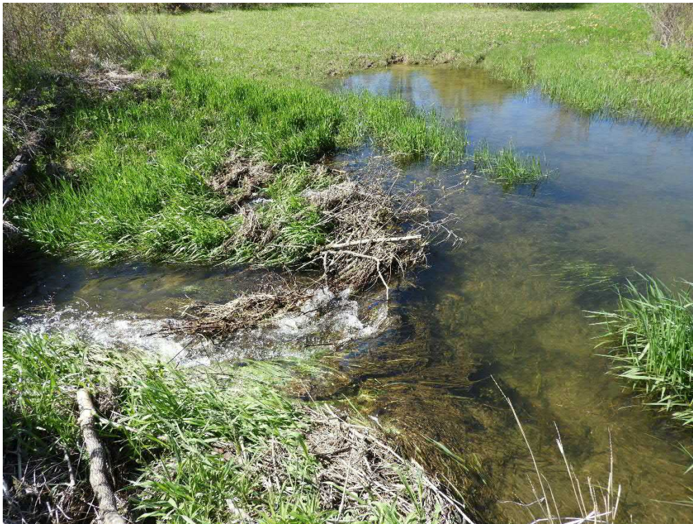
Photo 13: A beaver dam/debris within Harwood Creek directly downstream of one of the off-road vehicle crossings (right), which creates a potentially permanent barrier to fish migration. 12 May 2021.
