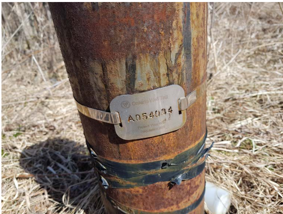
View of steel cased well at site.
