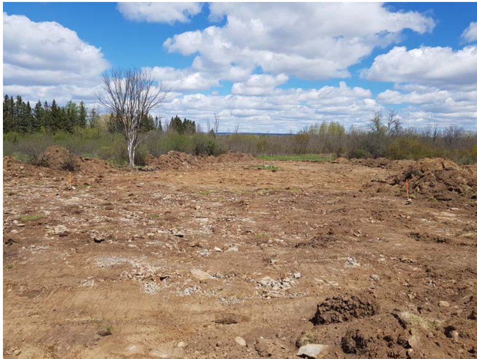
View of roadway construction after topsoil was stripped
