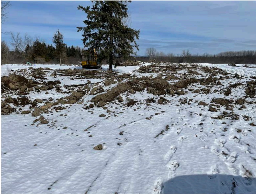
Front of site facing east
