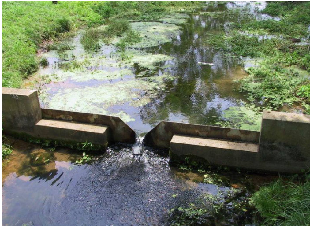
Figure 7-1: V-notch Cast-In-place Concrete Weir Wall Illustration
