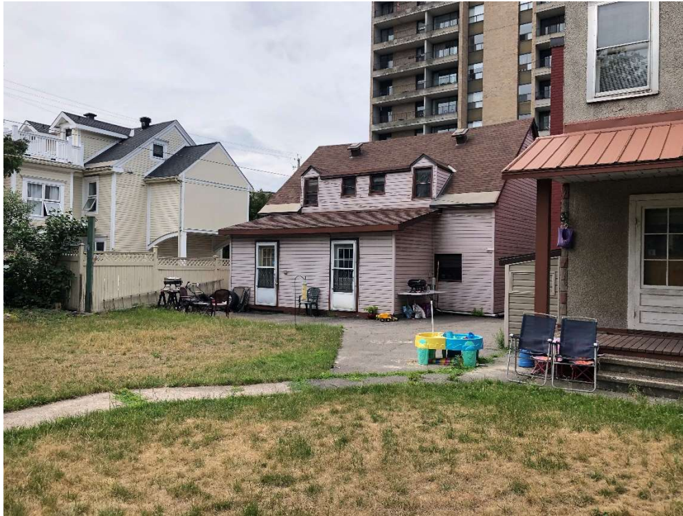
Photograph 1: Rear view of 113/115 Dalhousie Street.
